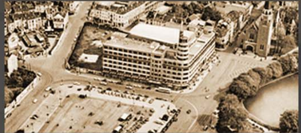
Place Flagey during its transformation, showing the "Ancien Institut National de Radiffusion" under construction. Photo: Collection Dexia Banque.
